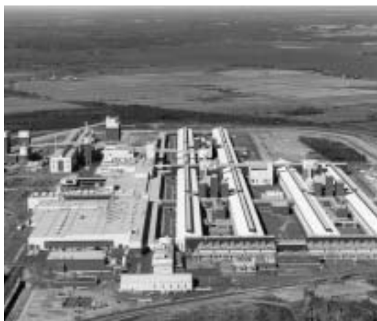
Alcan's new $2.6 billion smelter in Alma, Quebec includes a $180 million investment in the latest environmental technologies.
